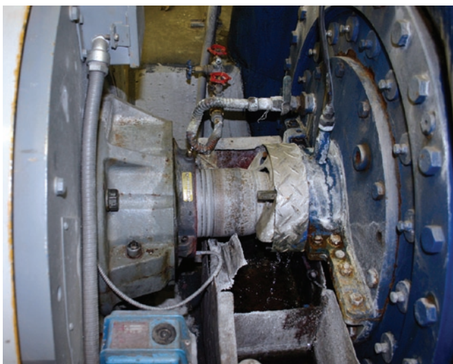
Cooper round flange in a trapped location
